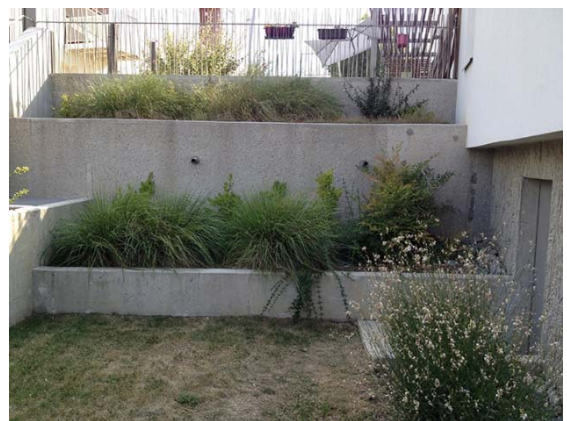
Fig.11. The carpark “green wall”
