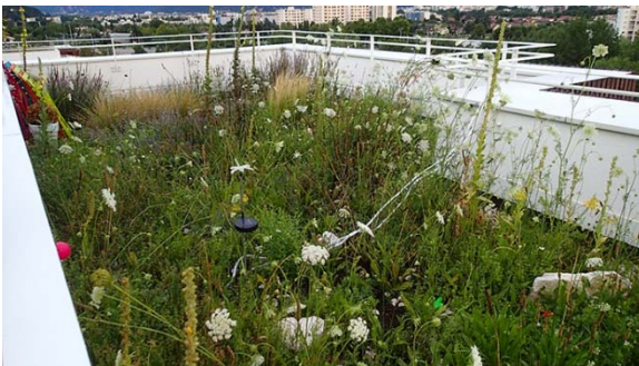
Fig.9. Extensive green roof after one year
