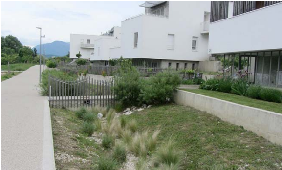
Fig.12. Wide planted gap separating private ground and public path rainwater dyke.
